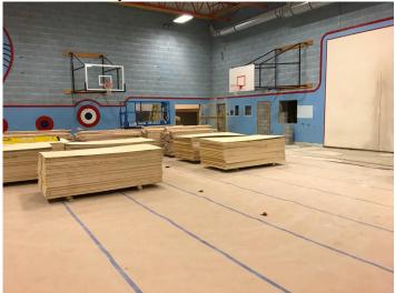
Work continues on the gymnasium. In this picture, you can see that a preliminary Top-Crete coating was added to the floor to smooth it. New holes for windows and doors have been cut. Heating, ventilation, electrical are all being upgraded. Sprinkler systems have been added. The floor has been delivered and is scheduled to be installed soon. Painting and additional deco coating are all due to be completed in the near future.
